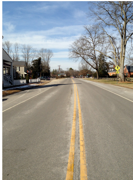
Figure 26. Route 301 in Hanover County
