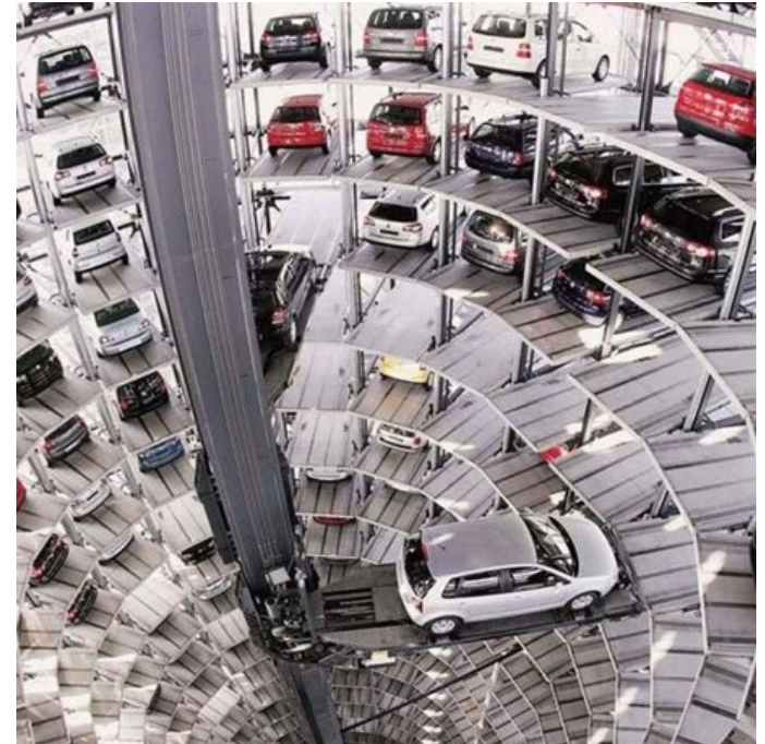
Fig. 2: A parking garage in Germany where vehicles are "retrieved"; takes up 80% less space than traditional American parking garage. (Source: Eilert, 2010)
