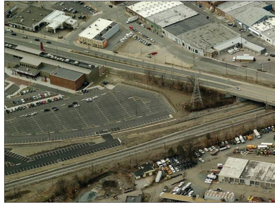
The current condition of the bridge
