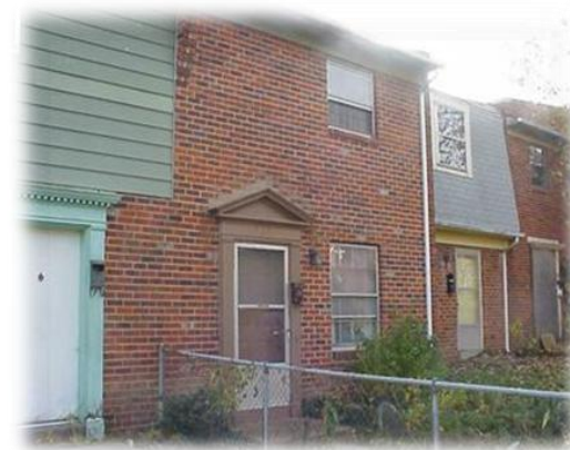
Photo 4.1.3: Homes in R-6 Zoning District Source: City of Richmond, Real Estate Assessor
